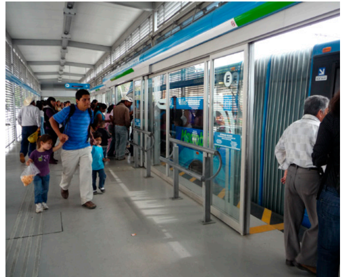
Figure 29: Barrier-free access to BRT bus in Mexico City. © Manfred Breithaupt, 2010
