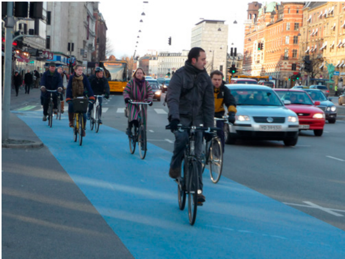
Figure 54: Painted cycling lanes at road intersections is an effective measure to improve the visibility of cyclists; Copenhagen.
