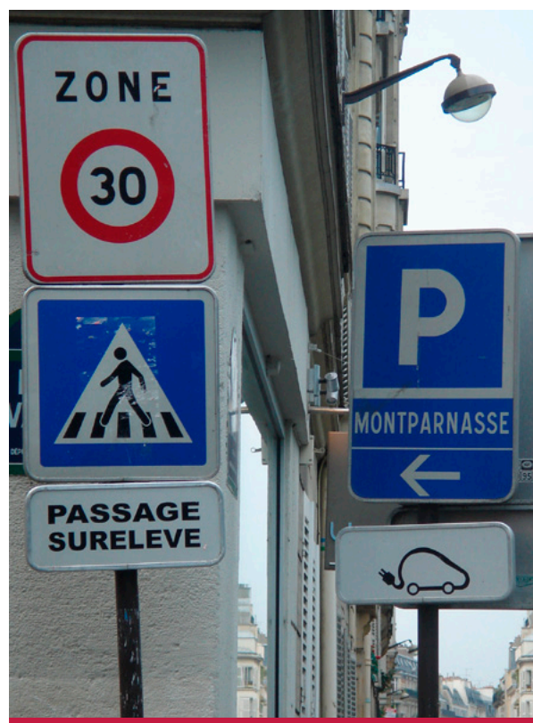
Fig. 22: Organising traffic in the inner city: traffic signs in Paris. ©Broaddus, Paris/France 2007
